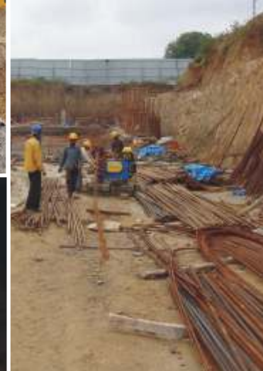
Reinforcement bar bending and butting, Station 13
