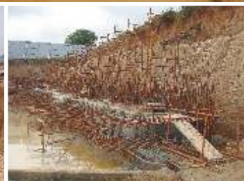
Reinforcement bar bending and butting, Station 13
